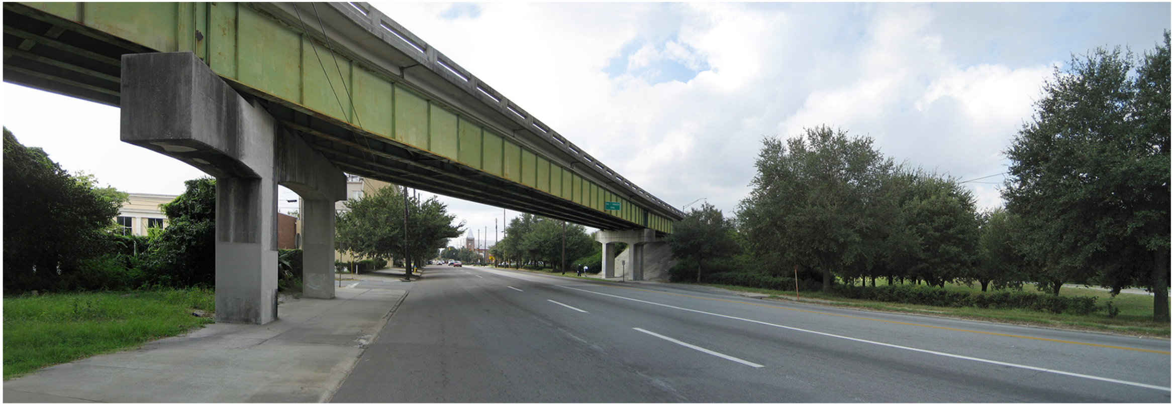
Current view of Martin Luther King, Jr. Boulevard and I-16 flyover.
