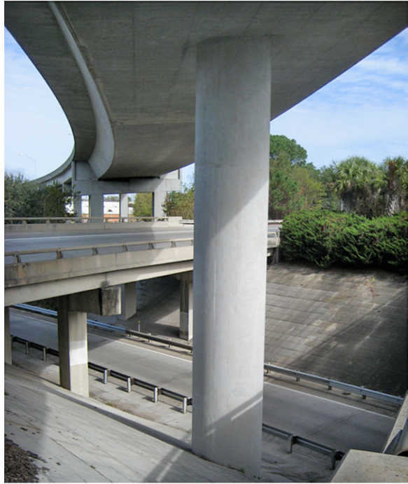
A newer elevated highway provides a high-speed connection to US-17 as well as an exit opportunity at Louisville Road, while allowing local surface streets to pass underneath.
